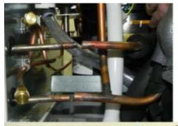
Once unit is recovered, unsolder Evaporator refrigerant lines
