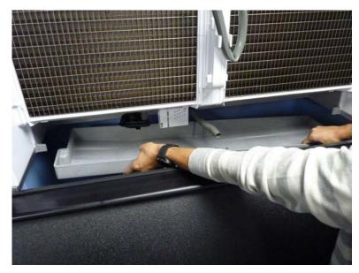
Slowly remove the sump from the bin so as to not hit and damage other components.
